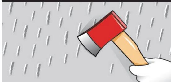
Hack uniformly across the wall (using a small axe, drill, or hammer) to create a rough and pitted texture on the surface. Clean the surface to ensure it is free from dirt and dust.
