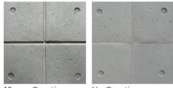
10 mm Grouting No Grouting
